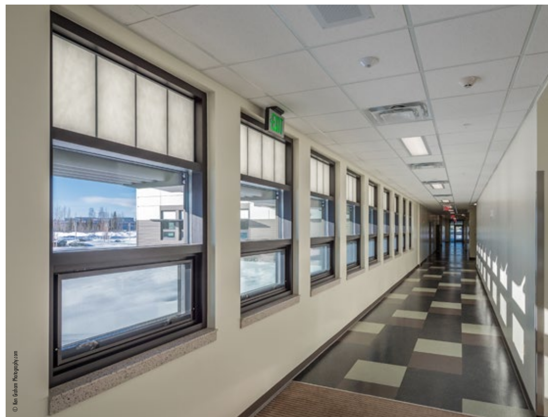
Left: Battalion HQ, Ft. Richardson, AK, Guardian 275 ® Translucent Adapter Panels Above: Close-up of a Guardian 275 ® Translucent Adapter Panel (TAP)
